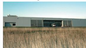
The reflecting glass façade optically hides the ground floor as continuation of the surroundings in a mirror image. The protruding office wing behind a black basalt concrete façade seems to hover over the landscape. Expanding façade parts associate CAMCOPTER® air vents and deeply framed windows create clear perspectives.
